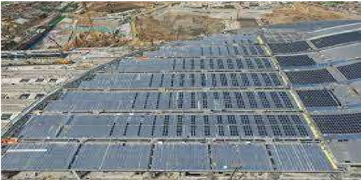
The roof of Asia's largest train station.
