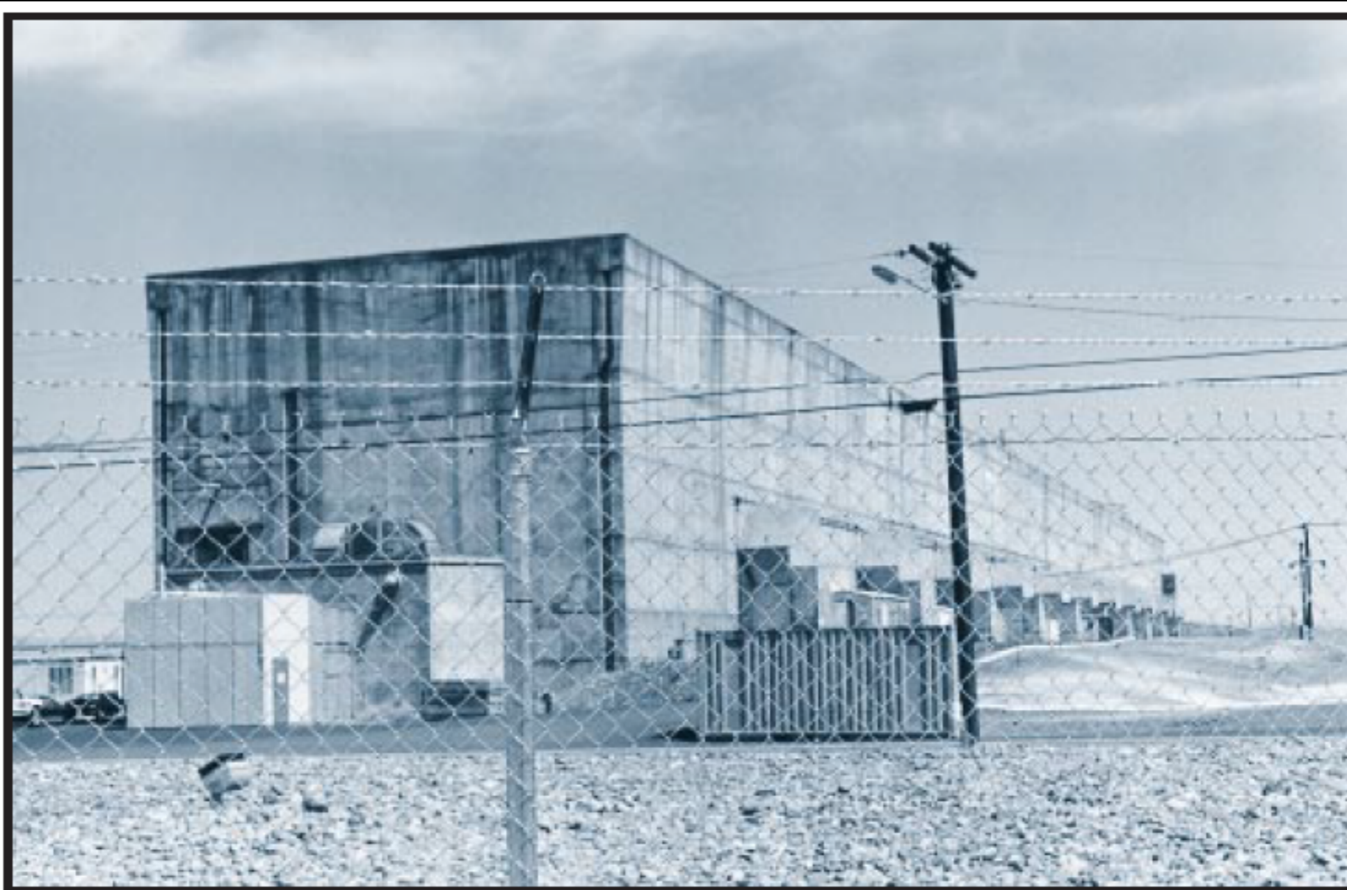
The T Plant was the world's first reprocessing canyon. In 1944, it dissolved spent fuel from the Hanford B Reactor and chemically extracted the plutonium, which was then used to form the core of the Trinity and Nagasaki bombs. It continued reprocessing until 1956. Today, the plant is used to decontaminate equipment. Hanford Site, Washington. July 11, 1994.
